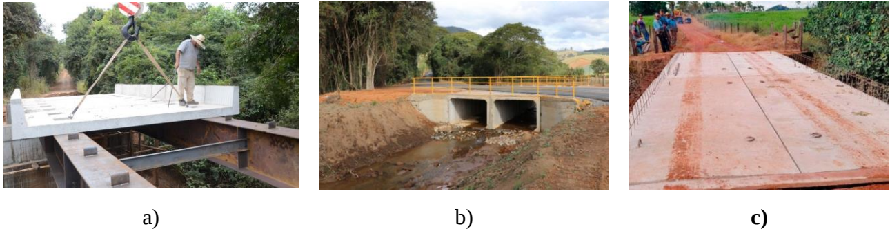
Figure 6 – Example of rural bridges commonly found in Brazil: a) prefabricated two-way slabs for a composite bridge [34] b) culvert bridge [35] and c) prefabricated deck slab [36].
