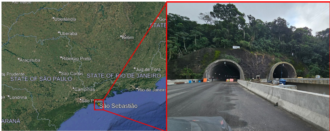
Fig. 17 Location of the underground highway tunnel under construction, in the city of São Sebastião, State of São Paulo, Brazil
