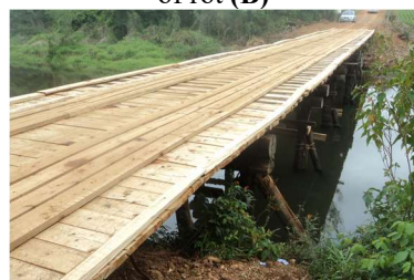
Absence of guardrails and wheel guards on the deck (E)
