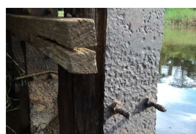
Use of metal connections without galvanization (C)
