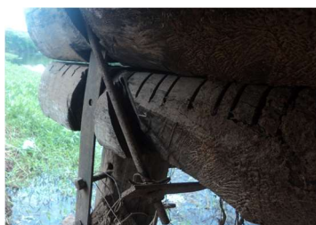
Presence of oxidation in the metal connecting joints (D)
