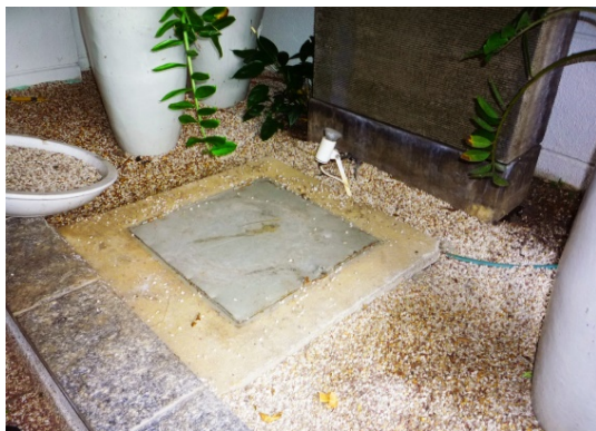
Figure 4 Access cover of the non-potable water reservoir
