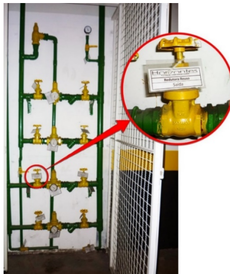
Figure 3 Pressure reducing station of non-potable water with the same color as that of the drinking water pipes
