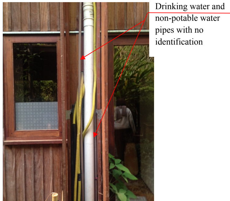
Figure 7 Inside a shaft with no identification that differentiates the pipe systems
