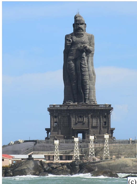
Figure 8. (a) Panoramic view of Vivekananda and Thiruvalluvar memorials constructed on monolithic charnockite islands situated at the meeting point of Indian Ocean, Bay of Bengal and Arabian Sea, (b) Vivekananda memorial constructed using polished blocks of charnockite and (c) the 41 m (133-feet) tall sculpture of Tamil poet Thiruvalluvar. The statue is made entirely of charnockite blocks.
