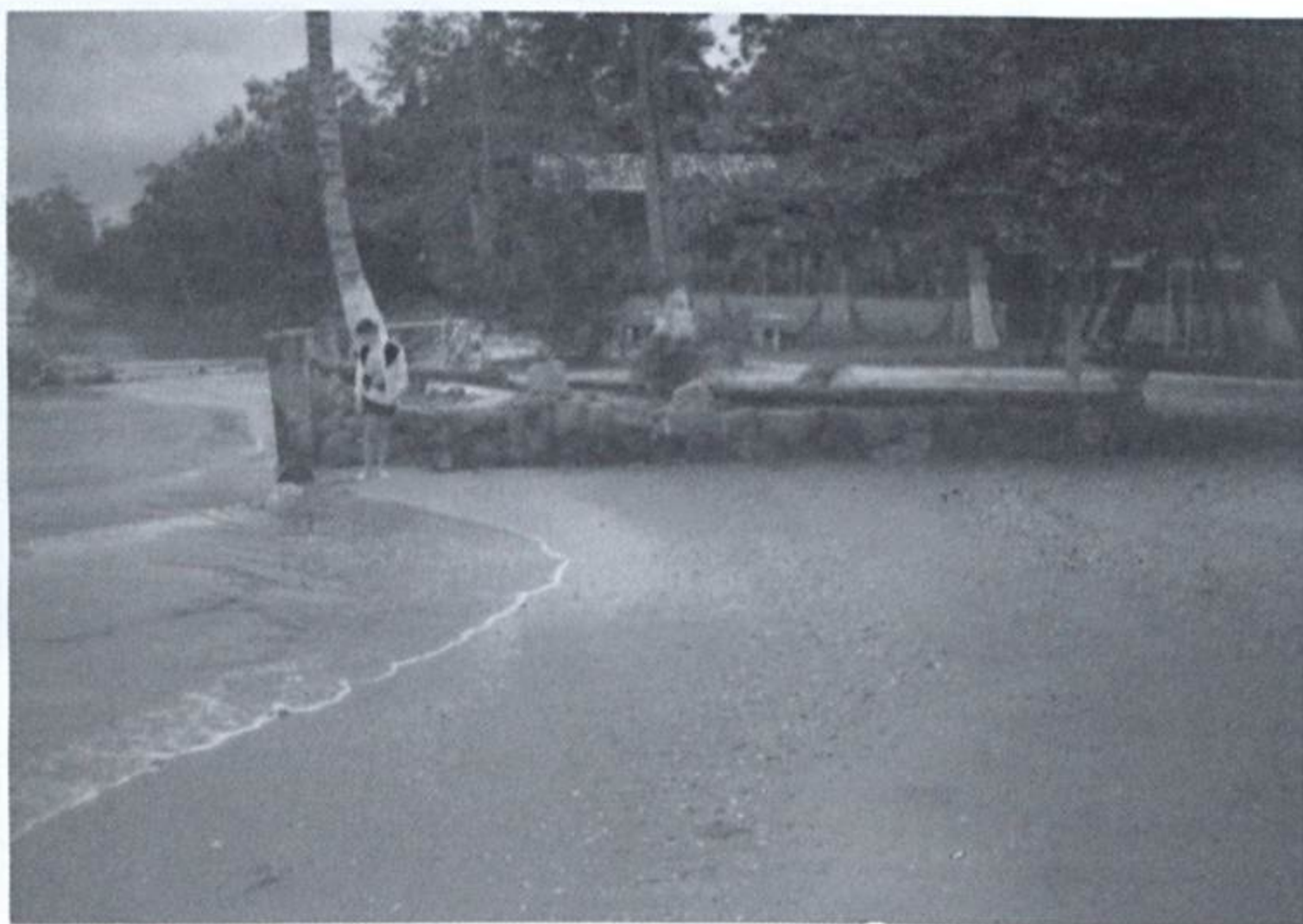
Fig. 14 — Erosion of a wall of a hotel built in the sixties, in the beach bordering the Caraguatatuba tidal flat (neap tide, may/1995).
