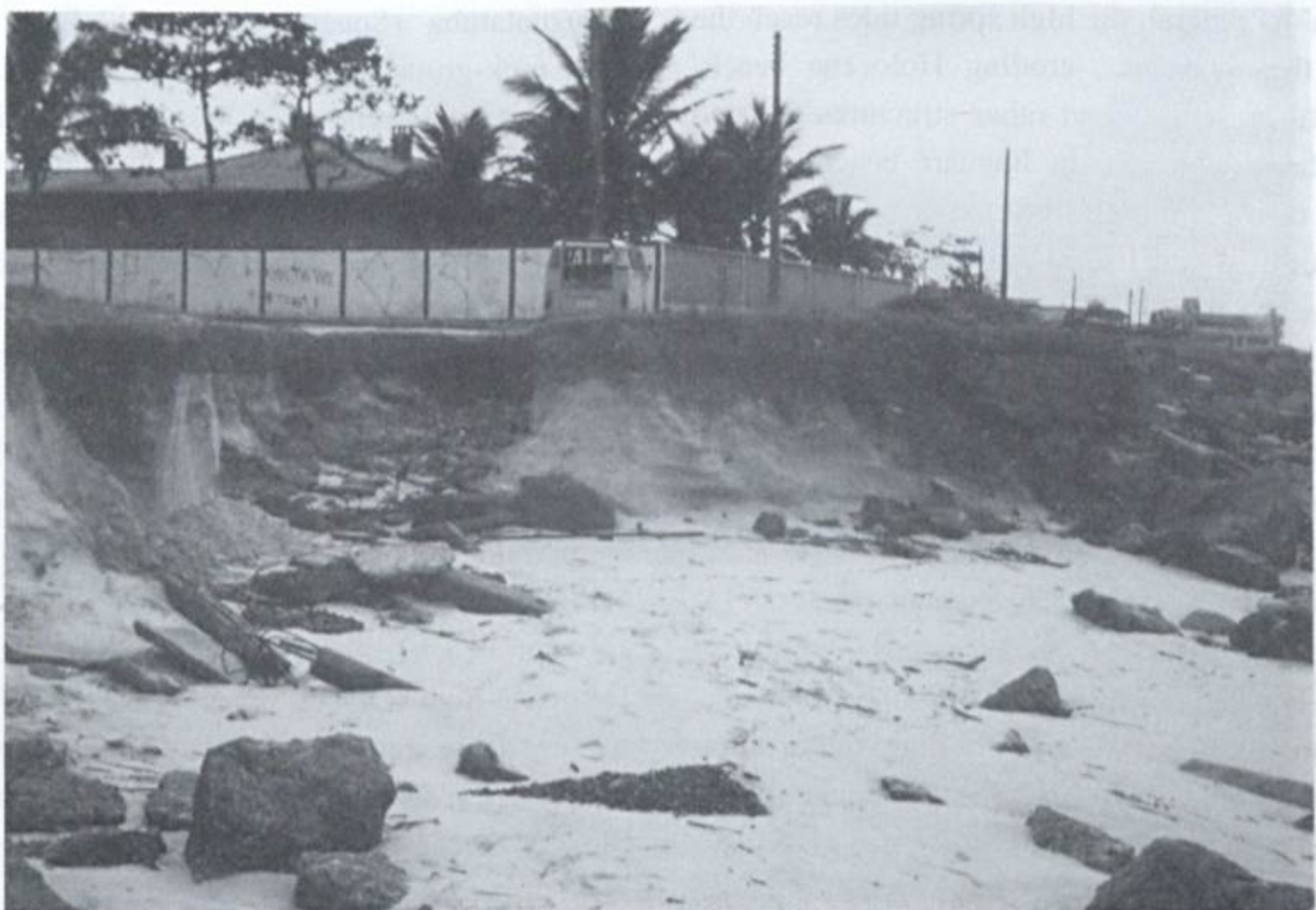
Fig. 10 — Erosion of uplifted Holocene marine terraces and street in the Itanhaém beach. Note rock-blocks put around the terrace to try to protect it against erosion (winter/1992).
