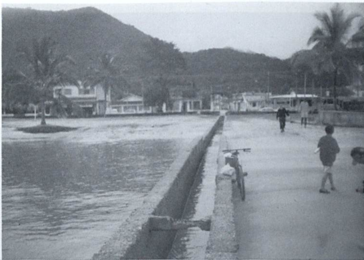
Fig. 13 — Erosion of the beach garden in urban center of Caraguatatuba and the impact due to construction of a new concrete jetty, causing strong erosion down-drift and deposition up-drift (neap tide, may/1995).
