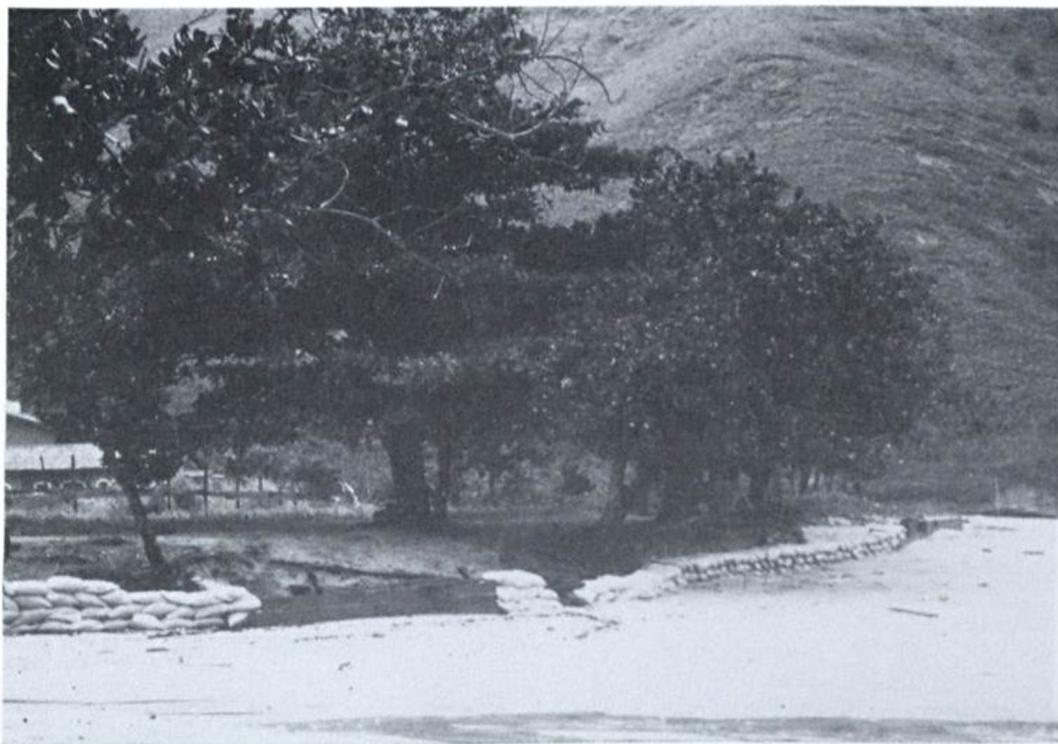
Fig. 12 — Erosion of Holocene beach-ridges, trees and a wall in the Guaecá beach (winter/1992). Mortar-bags were put around the wall to protect it against erosion. Some months later they have been destroyed.
