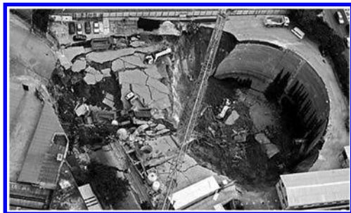
Figure 1. Tunnel collapse reaching the shaft.
