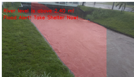
(c) The water level reaches the highest point of the floodwall. River level is computed as 2.40 meters.
