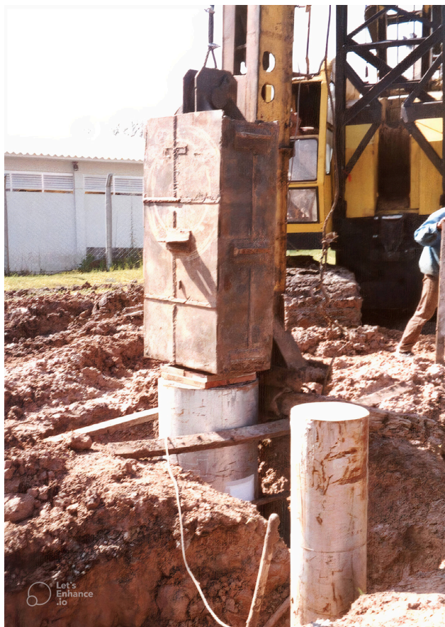
Figure 23. Hammer in PDA testing (Kormann, 2002).
