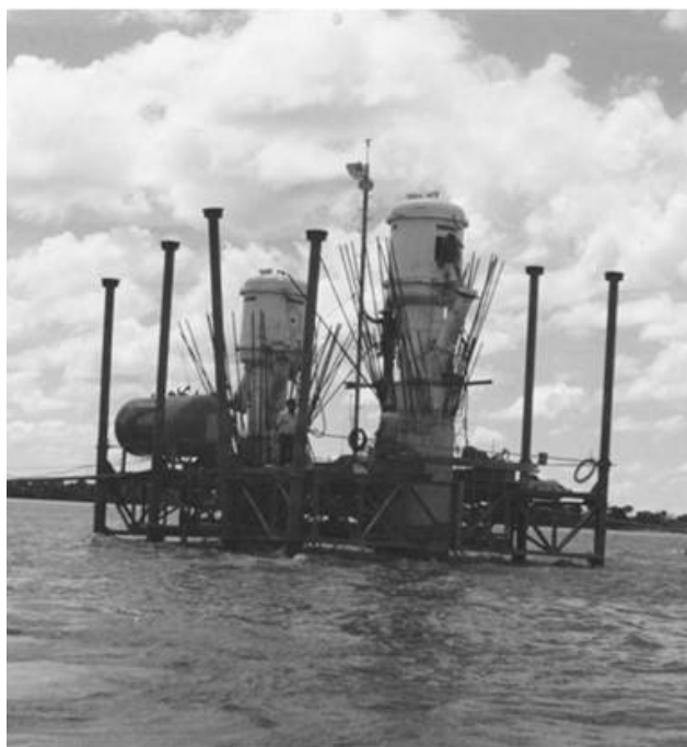
Figure 5. Example of pressurized drilled caisson platform and site work over a river in the interior part of Brazil (Source: Personal databank from the authors).
