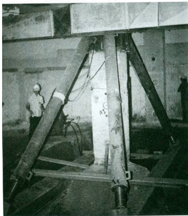
Figure 6. Foundation reinforcement at Paulista Mall (after Sayão, 2010).
