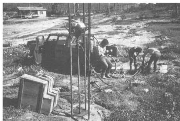
Figure 5: Drilling to monitor groundwater pollution due to industrial wastes, Taubate, São Paulo State.
