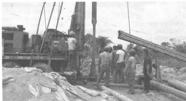
Figure 2: Drilling for water to be used for irrigation in the semi-arid zone, Bahia State.
