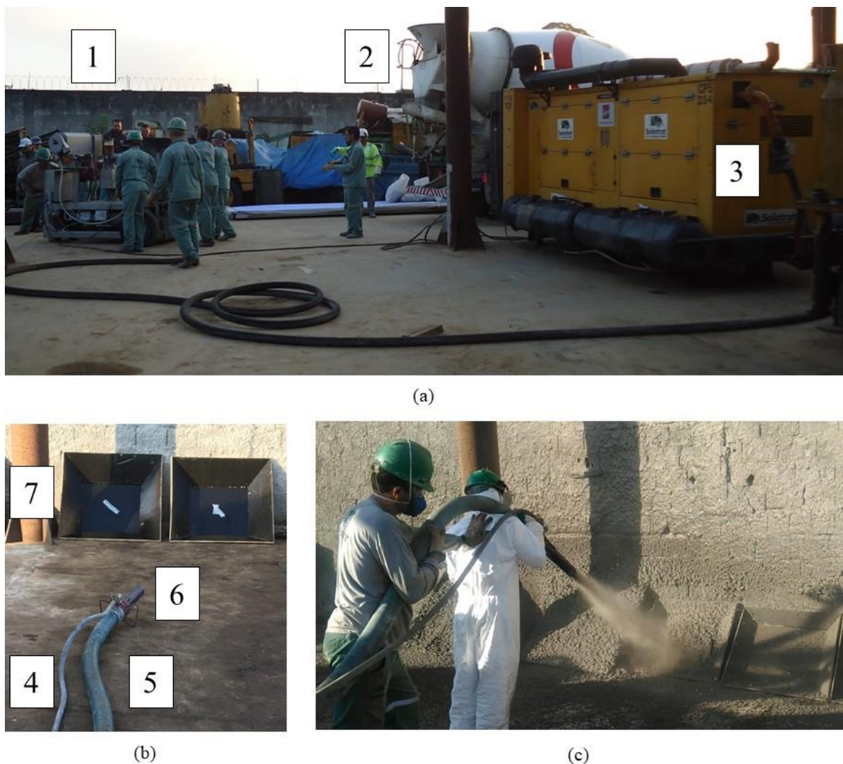
Figure 4 - Spraying process: organization of the process (a and b), concrete spraying process conducted by specialized nozzleman (c). Description of equipment: concrete spraying machine and accelerator pump (1), concrete mixer (2), air compressor (3), hose for accelerators (4), hose for concrete (5), nozzle (6), panels (7).
