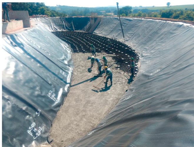
Fig. 2. The industrial water pond after being recuperated with a new HDPE geomembrane.
