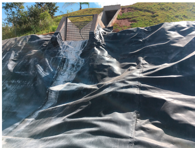
Fig. 1. The industrial water pond geomembrane before the exhumation, in service.
