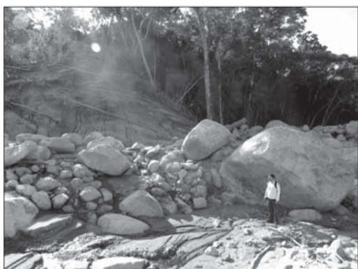
Figure 16. View of the levee formed in the left Guarda-Mão river bank.
