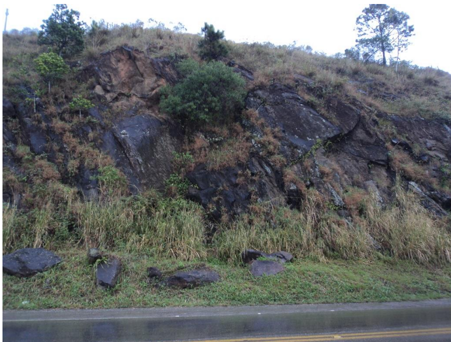
Figure 3. A slope at the beginning of the studied site. Notice the boulders at the slope's foot, and scars of failures in the rock slope, probably from rockfall events.
